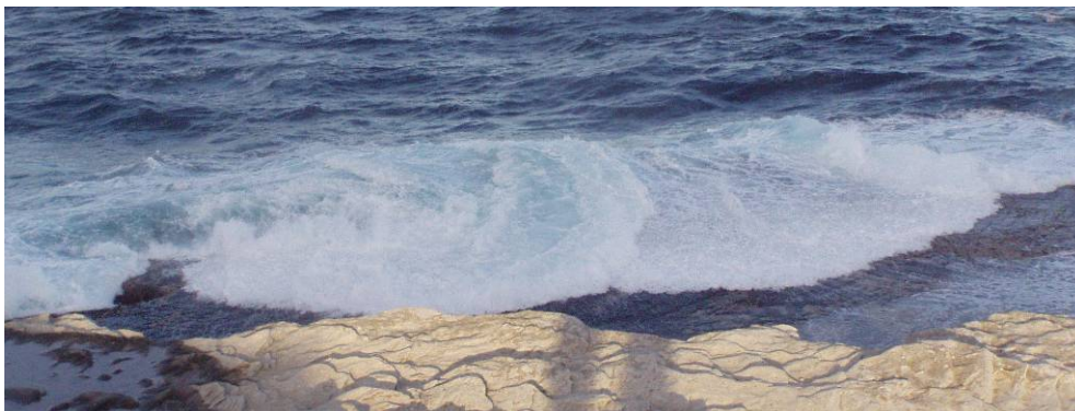
Photographs 4, 5, 6, 7: Overtopping at a popular fishing location at Jolong, north of Cape Banks
